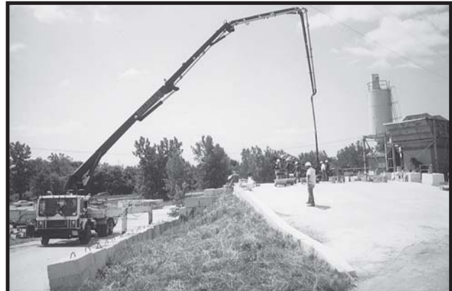
Figure 1: A vertical pump boom configuration can result in loss of entrained air in concrete
