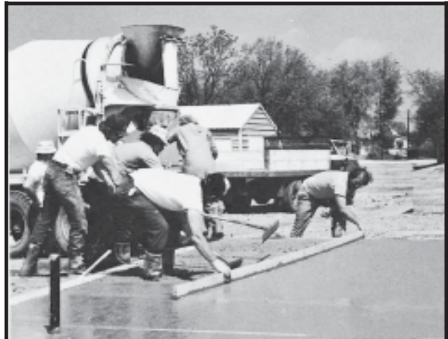
Finishing Concrete Flatwork
